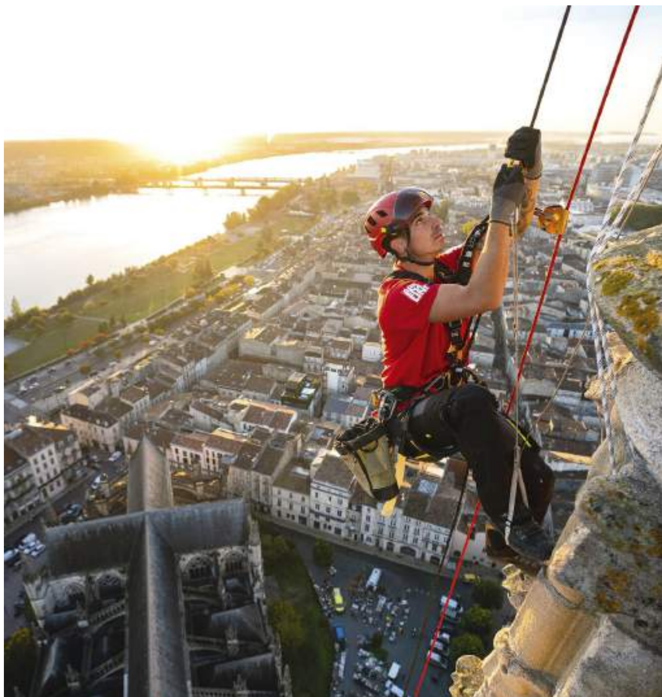
Installing monitors on the spire of the St Michel Church, Bordeaux, France © 2021 Petzl Distribution - Vuedici.org - Adréaline - Bordeaux City Hall
